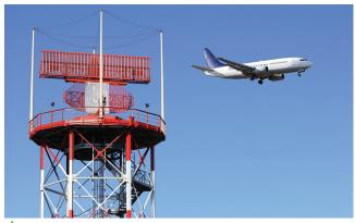
▲ Fig. 2 Airport co-located primary and secondary radar system. The SSR radar antenna is at the top with the S-Band antenna immediately beneath it. (Photo courtesy of Shutterstock.com).
